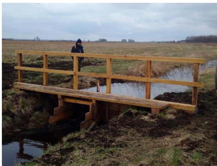
Figure 2. Wooden dyke built to block an old draining ditch as part of the rewetting project to raise water levels and restore fen habitat for Aquatic warbler with a climate mitigation benefit. Near Krychów, Poland. April, 2022. Photo by Sviataslau Valasiuk
